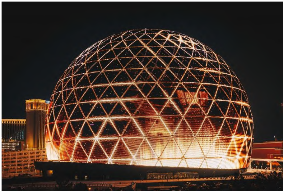
Sphere's exterior – the Exosphere – is fitted with 1.2 million LED pucks and is fully programmable. Photo: Sphere Entertainment
